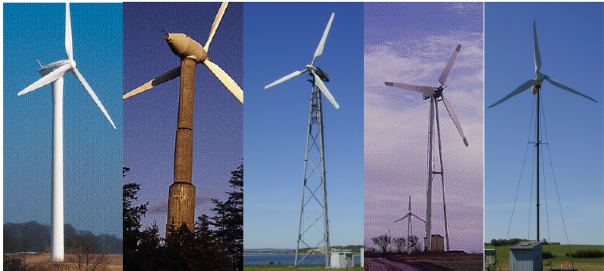
Figure 7-1. Various tower structures. From www.windpower.org , © Danish Wind Turbine Manufacturers Association.
