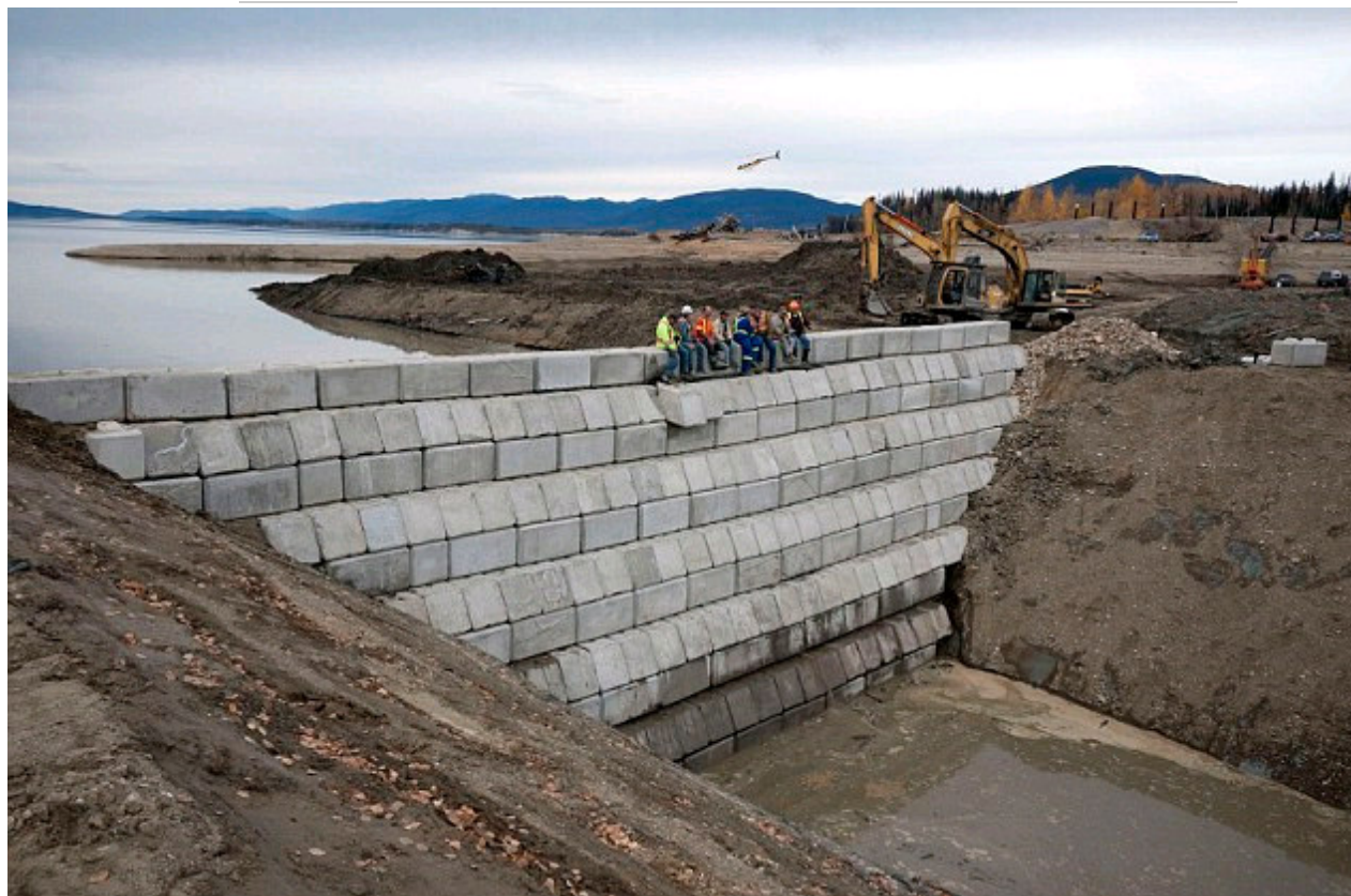
Before: The make-shift dam was made of concrete and was 130ft wide and 30ft high
