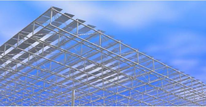
Fig. 2: Close view of the roof covered with PVP.
